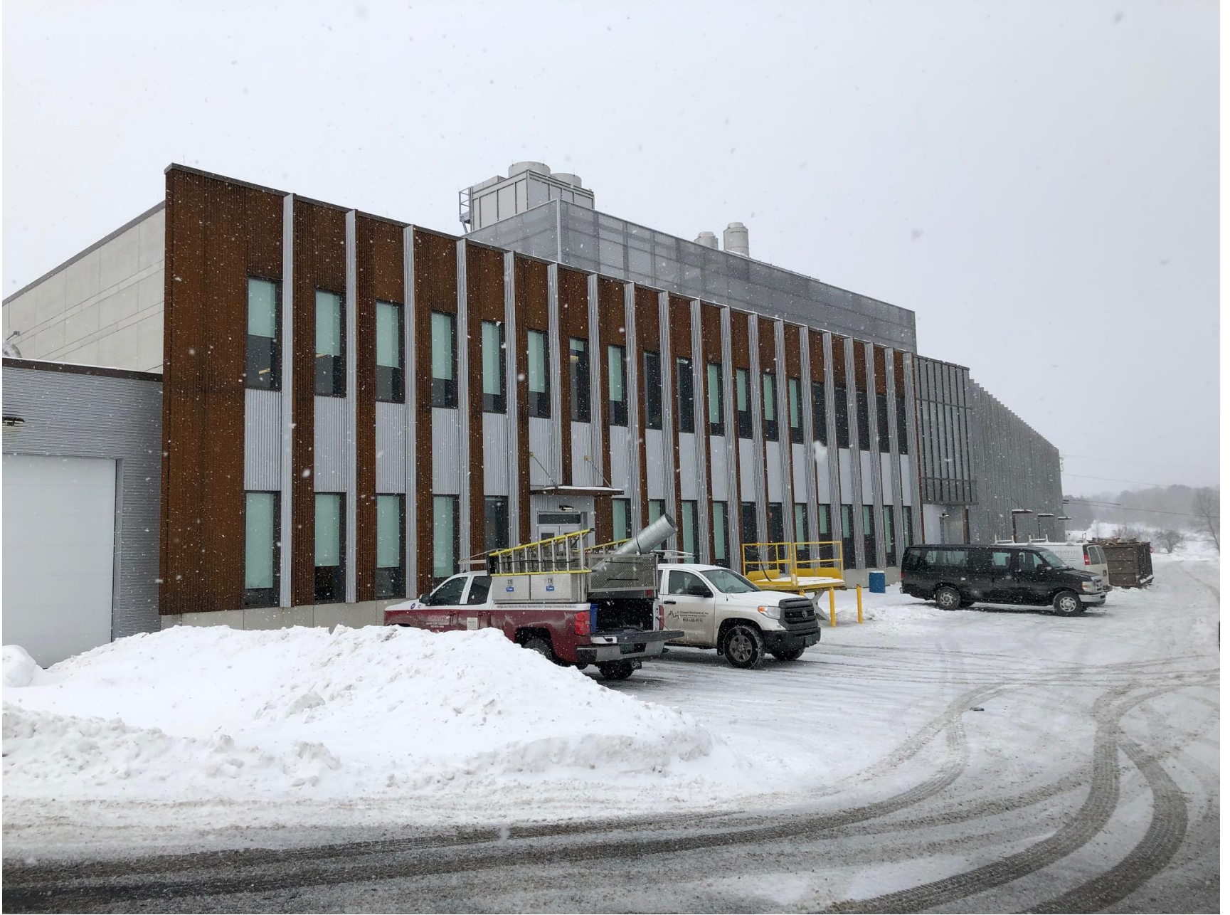
Lower Level Looking North 11
